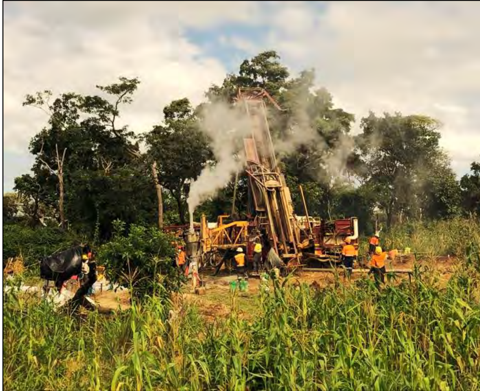
Figure 10-1 Drilling at Koné in 2013
