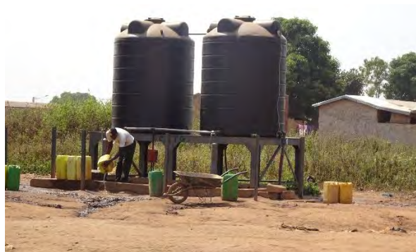
Figure 20-3: Water Tanks at Fadiadougou
